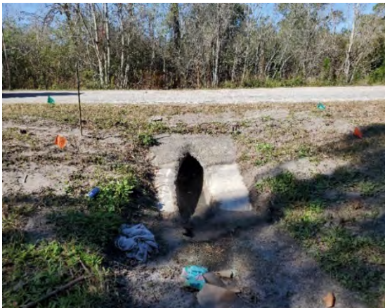
Figure 3-6 Existing Cross Drain, CD #1
