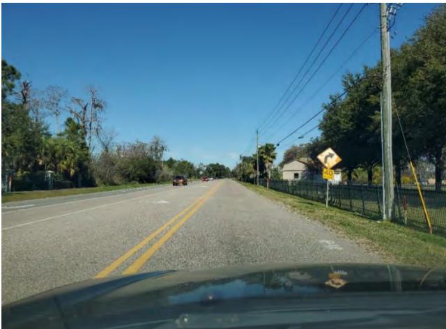
Figure 3-8 Roadway Facing North
