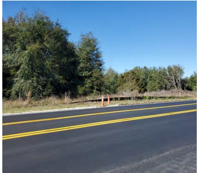
Figure 3-10 Roadside Facing North Near Hartzog Road
