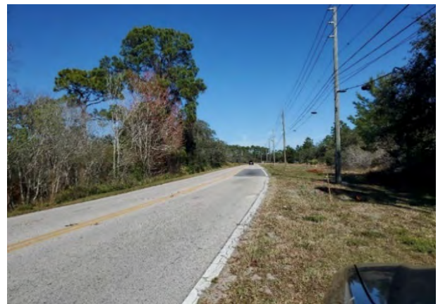
Figure 3-7 Roadside Ditch Facing North
