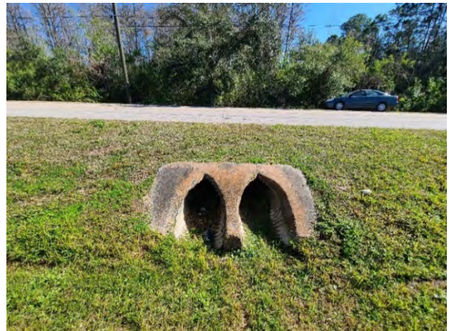
Figure 3-9 Existing Cross Drain (CD #3)
